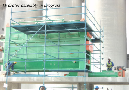
Hydrator assembly in progress
