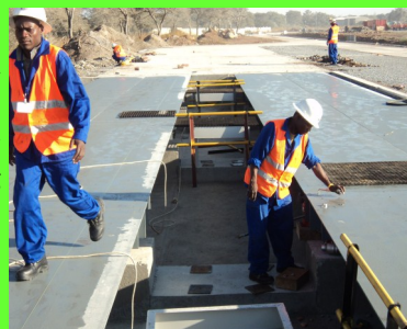
Weighbridges installation progress...
